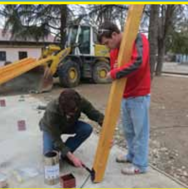
Jacob Buckwalter '14 and Bradley Wilcox '16 cementing in a post for the main support of the classroom.
